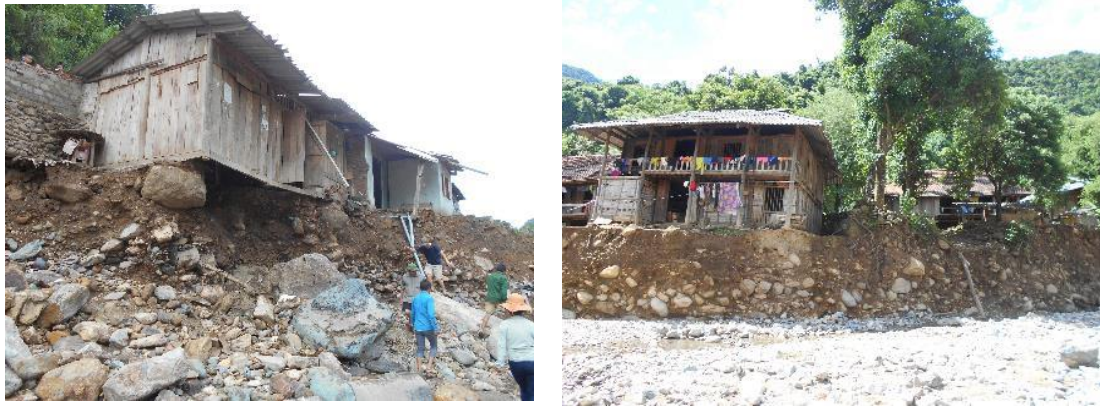
Figure 5. The land below damaged houses and land exposed by side erosion contains big rocks.
