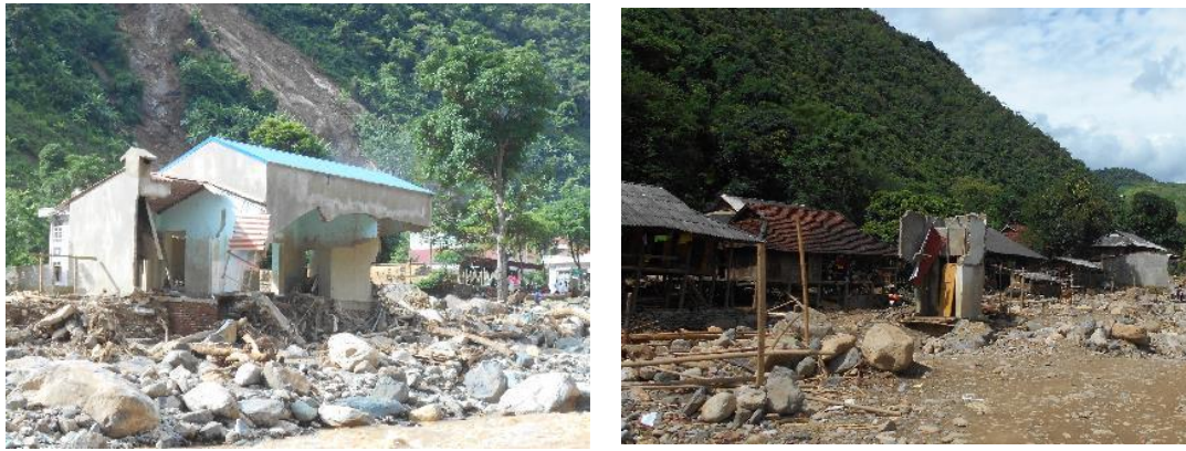
Figure 3. Many houses and building were swept away or destroyed.
